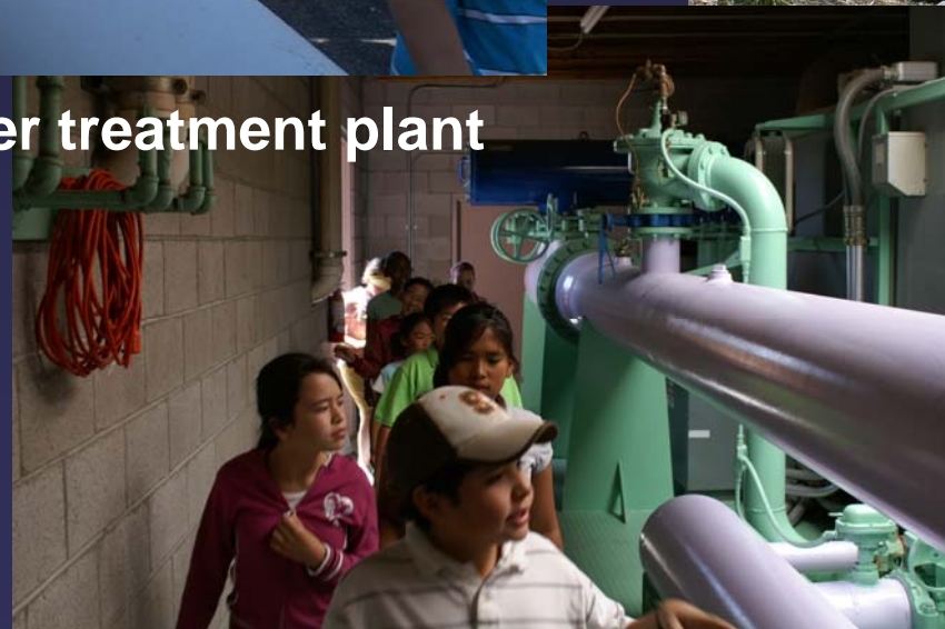
In the pumphouse
